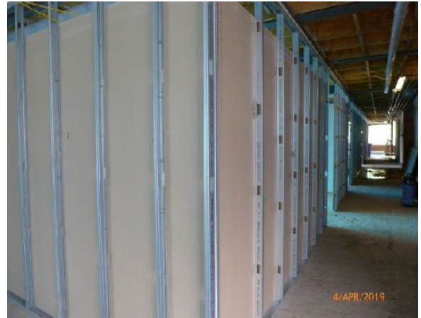
New Offices: General view of corridor looking West.
