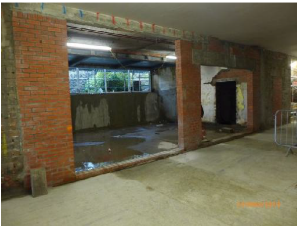
Lower GF - General views of shop front and floor space.
