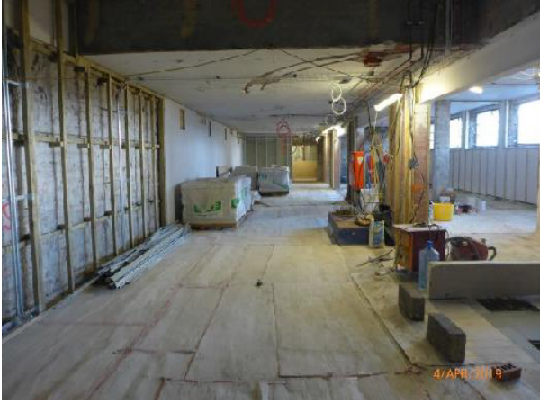
Lower GF – New Exhibition area – looking North.
