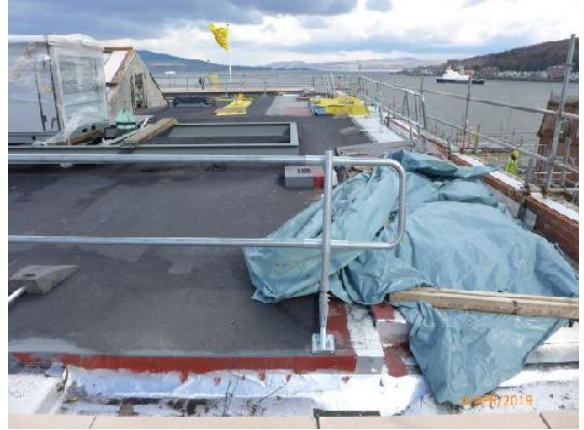
Looking East: General view: South area looking East.
