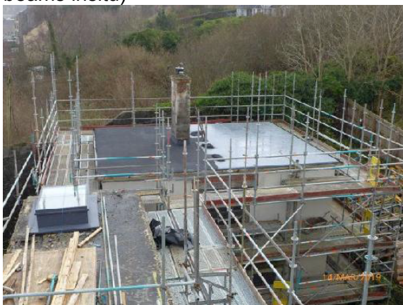
General View (Looking south): Caretakers House Roof.
