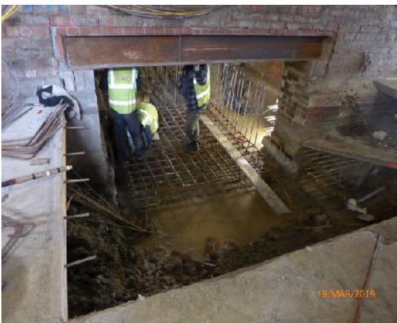
New Lift Shaft - Main Entrance Foyer / Circulation area / Undercroft – Reinforcement for the lift base in progress.
