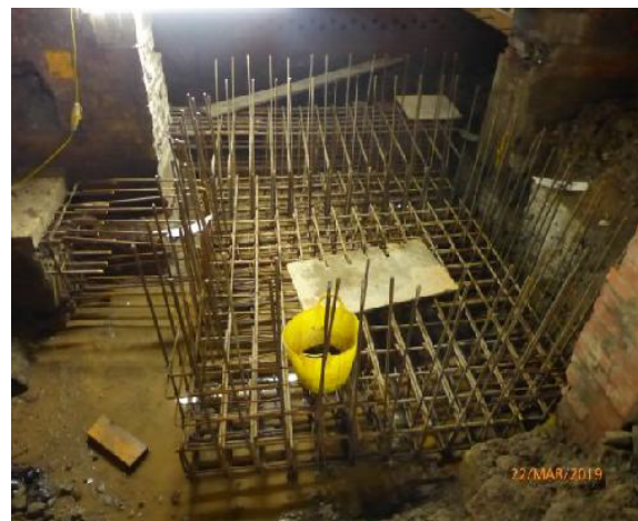
New Lift Shaft - Main Entrance Foyer / Circulation area / Undercroft – Reinforcement for the lift base in progress.
