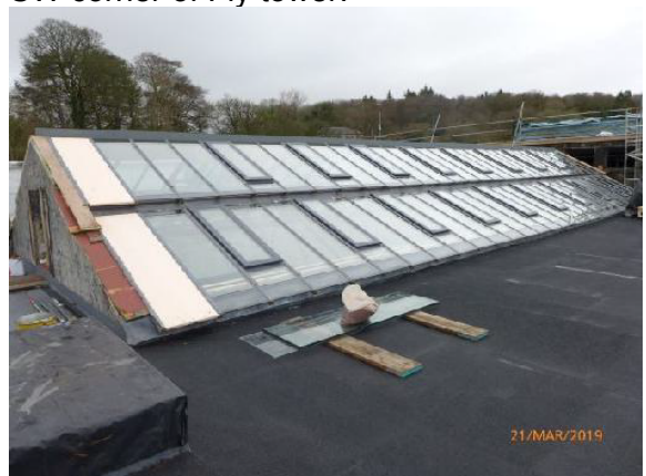
Roof light (looking North): new Glazing is substantially complete (NB: South and North end glazing panels & ridge roll awaiting installation).
