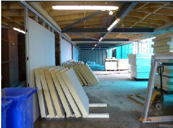
New Offices: General view looking East (stud partitions insitu).
